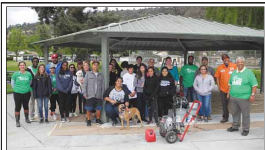
About 60 volunteers from the neighborhood, along with volunteers from Cal Poly University Pomona and several Pomona public works employees, pitched in to paint the inside of the gazebo in Westmont Park for this year's Pomona Beautification Day, under the direction of project leader Jorge Gajeda, at right. The group also cleaned up tables and benches in the park. See more pictures on pg. 8.
