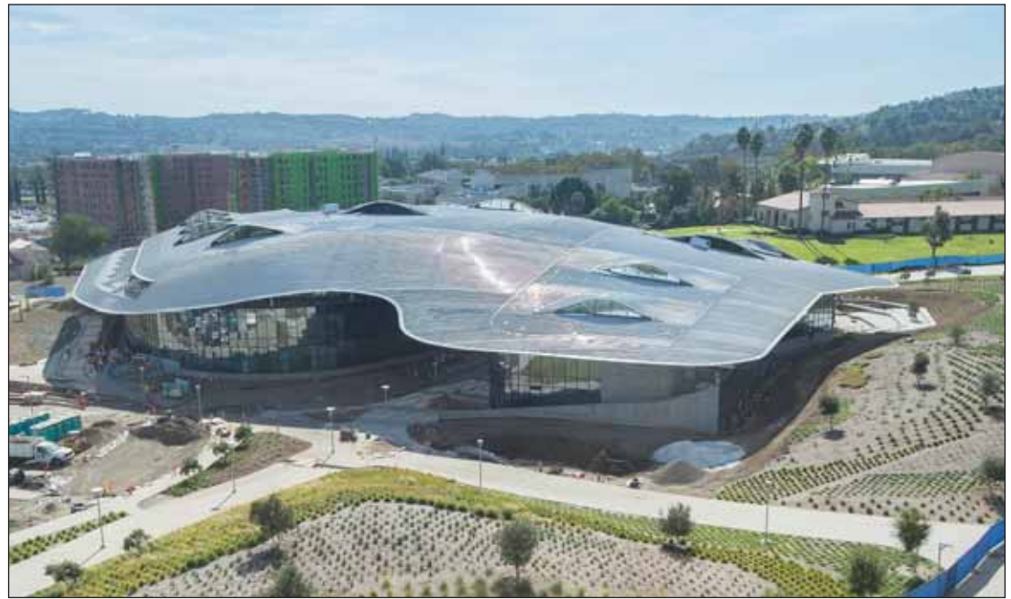
An aerial photograph highlights the design features of Cal Poly University Pomona’s new $79 million student services building.
