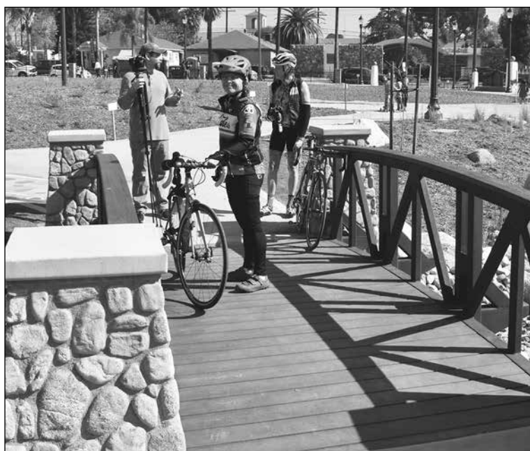
One of two bridges in the new Phil and Nell Soto Park was already in use on opening day.
