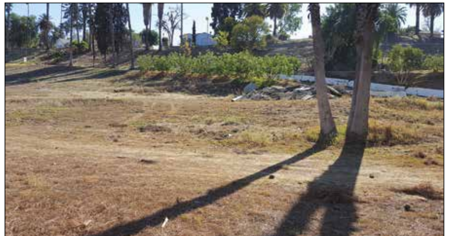
Fairways have browned out and concrete debris is piled high (at rear) during a refurbishment project under way for the past four years at Palm Lake Golf Course in Pomona.
