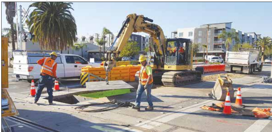
Workers place a steel plate over an open underground vault in the “slow lane” of Garey Avenue in Pomona as work gets under way preparing for the Gold Line tracks reconfiguration project.
